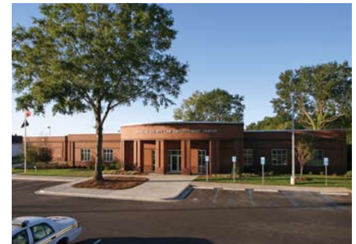
kershaw county law enforcement center
